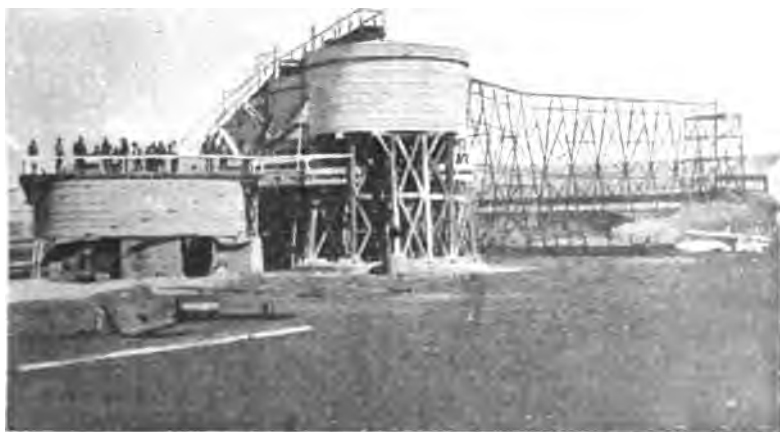
FIG. 147.—TANK FOUNDATIONS.
